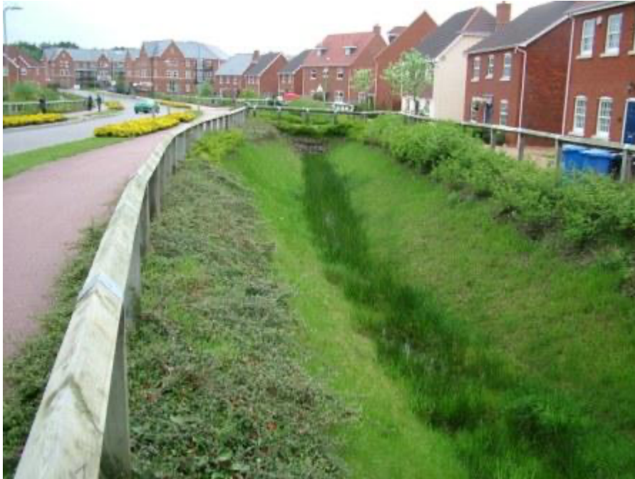
Figure 1: A sustainable urban drainage (SUD) scheme as part of a new housing development in Cambridge* [Alt text: Photo of grassy swale, showing development of wet grassland vegetation in its base, sandwiched between a road and a row of houses.]
