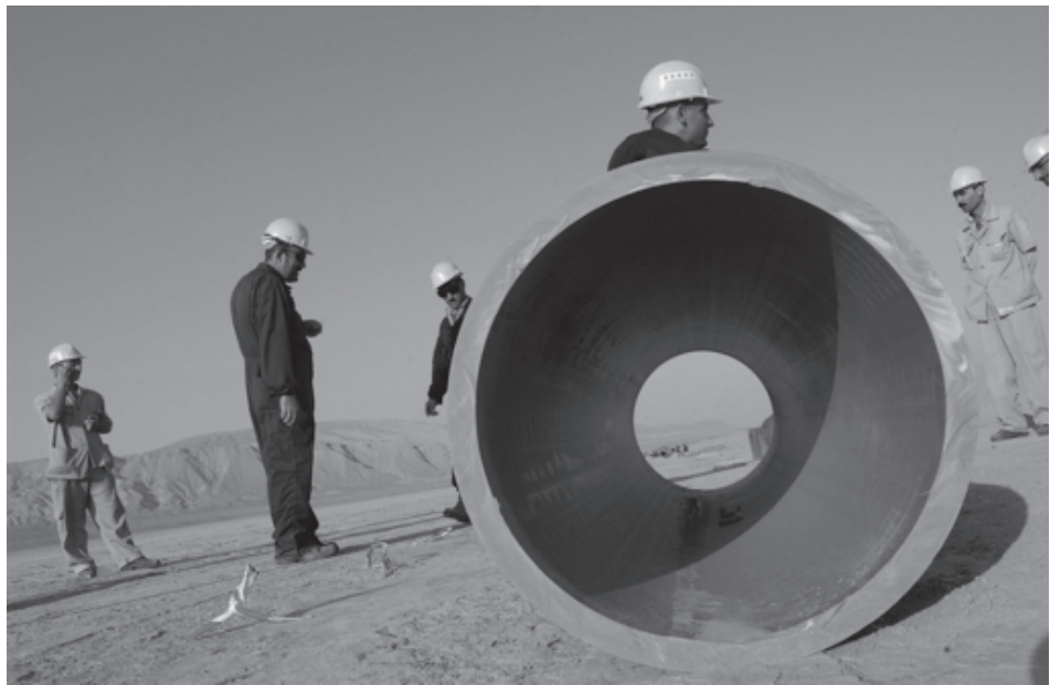
Oil pipeline construction, Azerbaijan.
