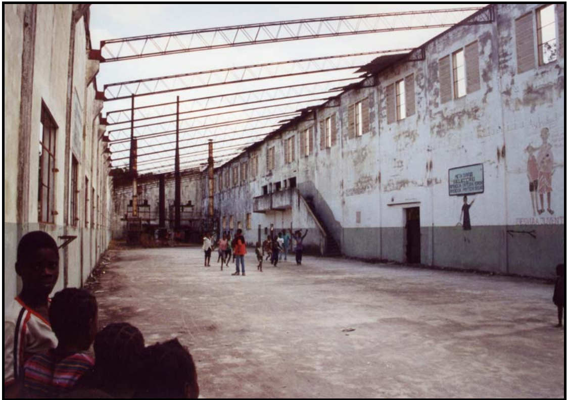
Figure 4.4 Destroyed cashew factory in Namacurra
